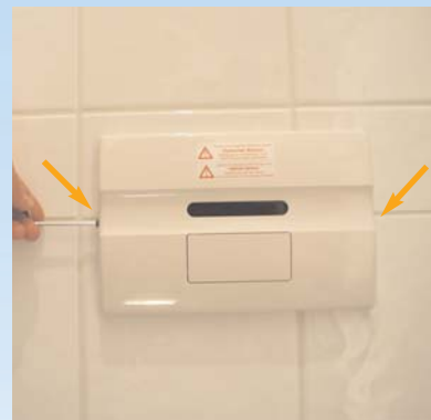
Install front panel and fix it with the safety screws on both sides.
